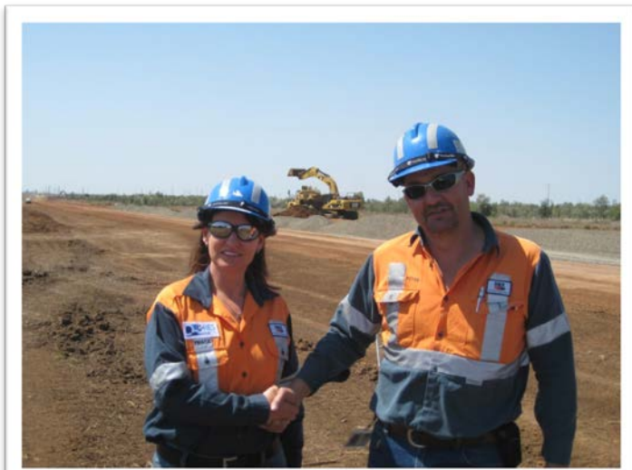
PHOTO: First work package awarded through the BMA Local Buying Program – BMA Blackwater Mine “BMA’s Peter Fuller and Community Development Supervisor, C-Res Tracey Cuttriss-Smith with a significant gravel road base order”
